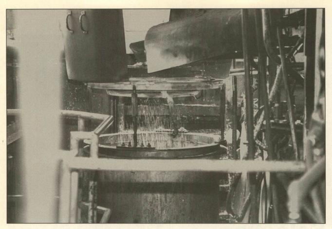
Molten lead is poured through a droplet-forming and sizing screen in the shot tower.
